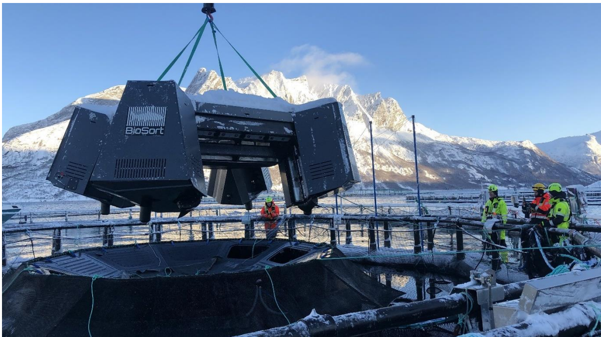
Figure 9 Photo of the installation of the Dome sensor housing to iFarm 1 (M10).
