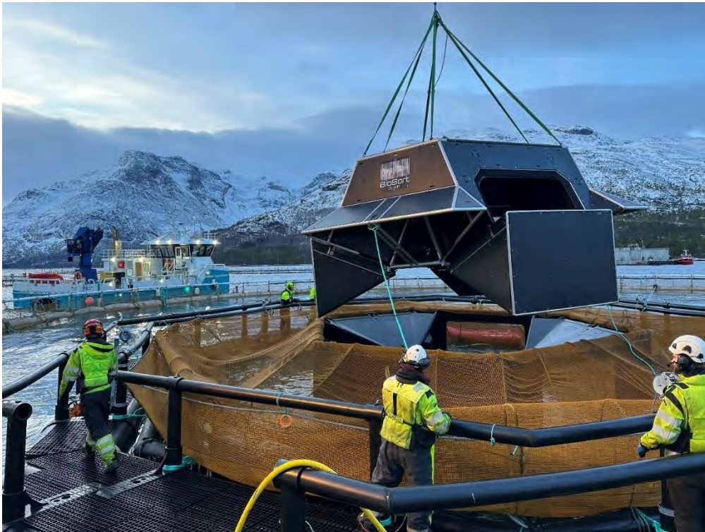
Figure 12 showing the iFarm house installed in Hellarvika cage M3.
