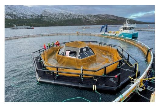
Figure 13 showing the iFarm house with one sensor unit (visible with lights) and two dummy openings being installed in cage M3.
