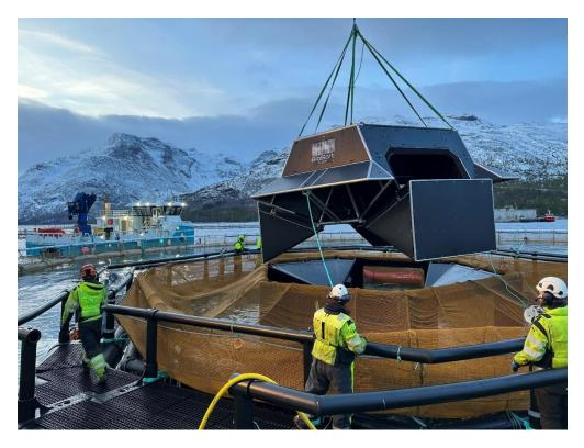
Figure 12 showing the iFarm house with one sensor unit and two dummy openings installed in Hellarvika cage M3.
